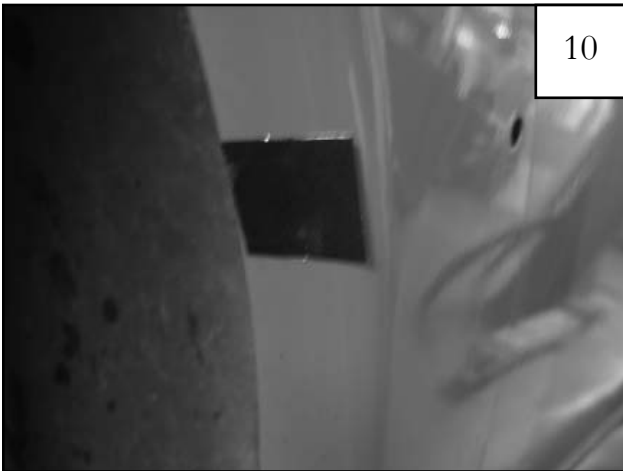
Install a Tab (MT1-0002) centered over mark made in Step 9. Edge of Tab should be even with edge of sheet metal.
