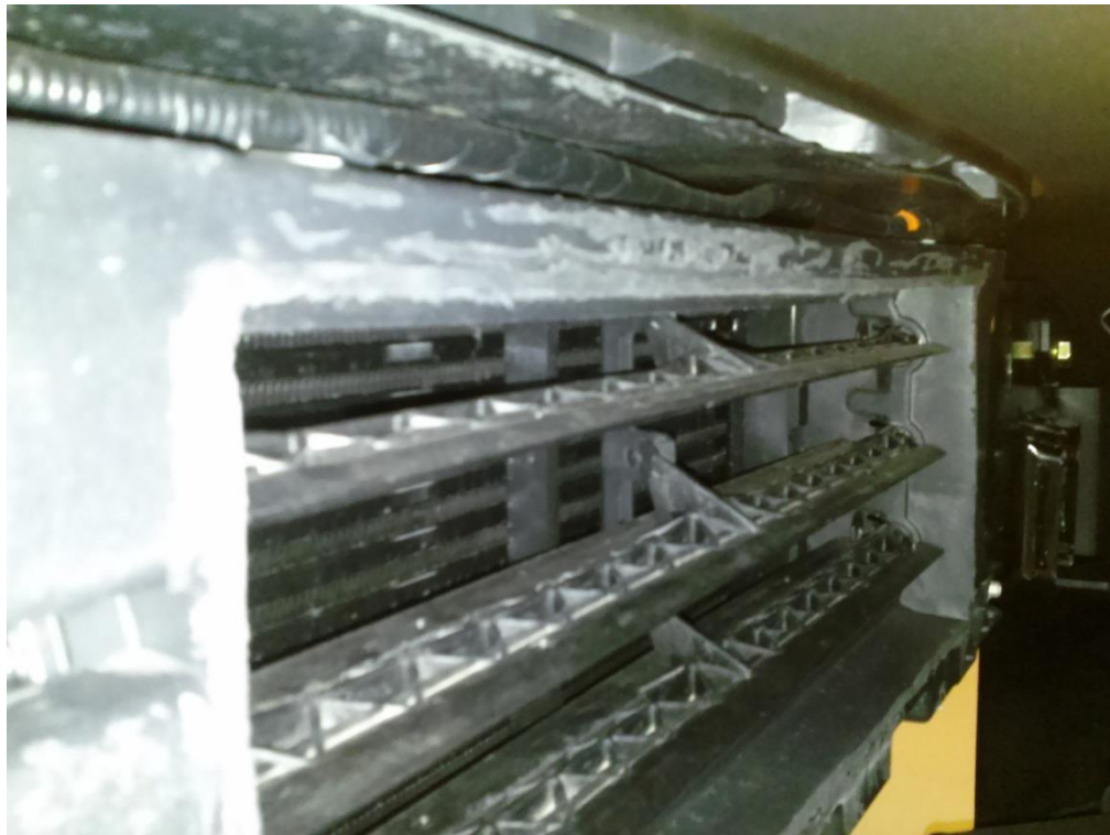
Figure 4 (Louver w/ shroud cut away at base)
