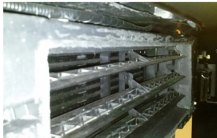
Figure 4 (Louver w/ shroud cut away at base)
