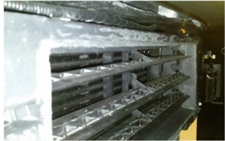
Figure 4 (Louver w/ shroud cut away at base)
